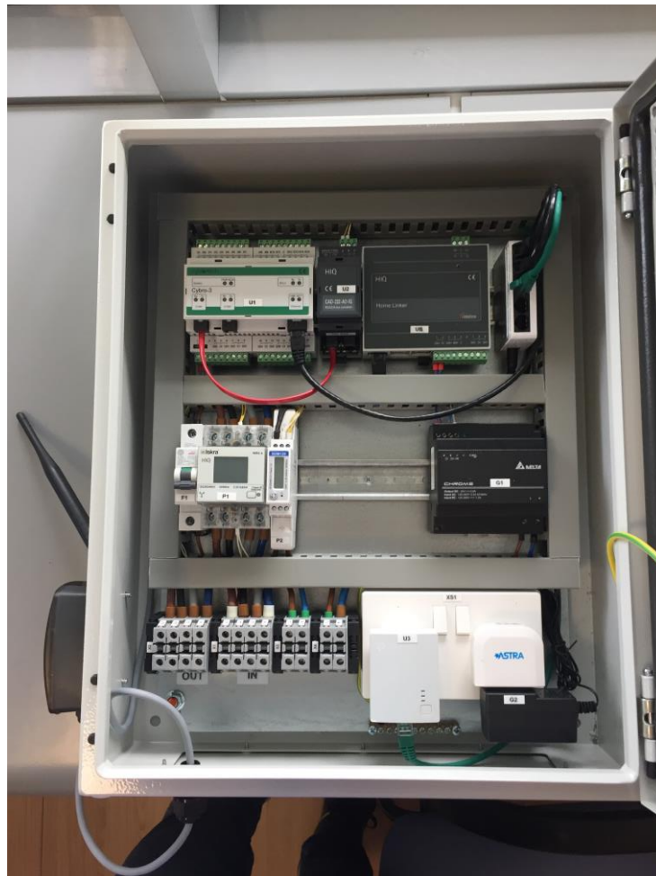
Figure 10 HEMS controller installed in dedicated panel
