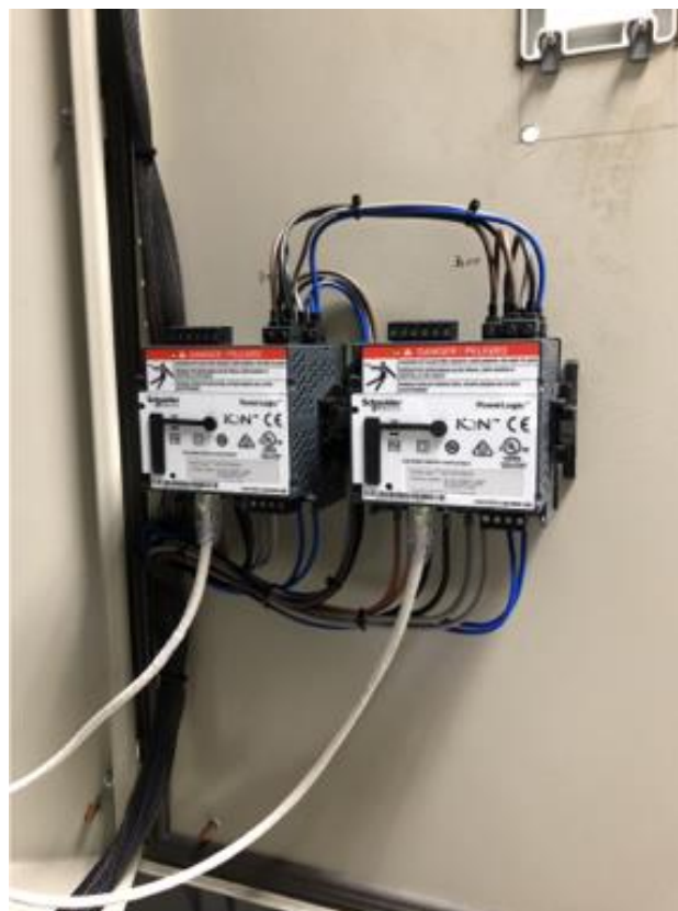
Figure 8 Installed Smart Meters in the University Campus
